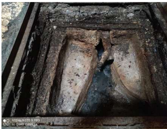
Fig. 1. A junction of a free-flowing drainage conduits inside a manhole.
